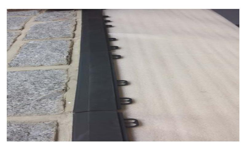
Starting at the front right corner, lay the first row of tiles, connecting with the female edge pieces as you go, and repeat this process, making your way backwards.
