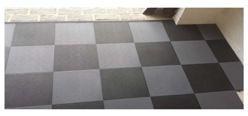
At walls, cut tiles to size, ensuring that an adequate expansion gap is left (around 8-10mm)
